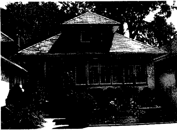
Figure 1: 7641 South Merrill Avenue
